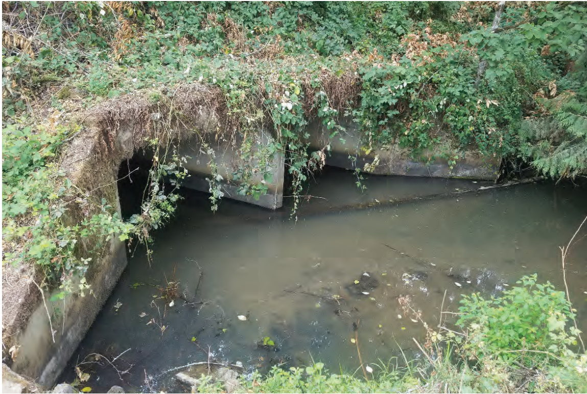
Figure 11: View of the twin box culvert. Wet passage likely provided, but no dry passage available.
