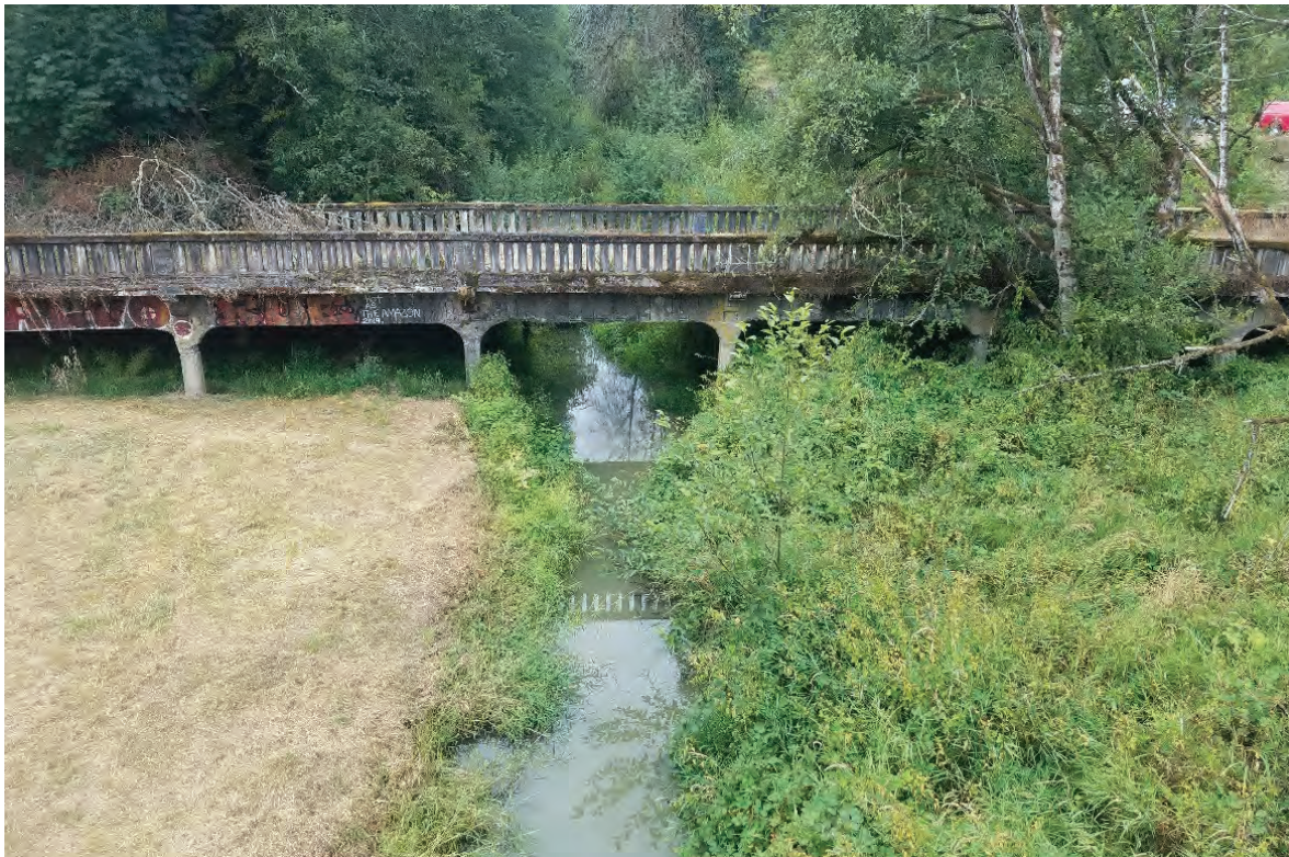
Figure 18: View of McCarthy Creek and old Highway 30 bridge. Passage is provided below old Highway 30 but could be improved. Riparian area deteriorates in proximity to Highway 30. Traffic on Cornelius Pass Road is visible in the upper right of photo.
