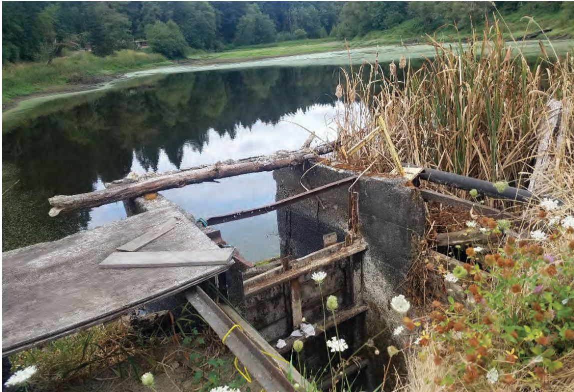
Figure 13: View of the riparian conditions above the twin box culvert. Highway is a barrier to wildlife at this location.
