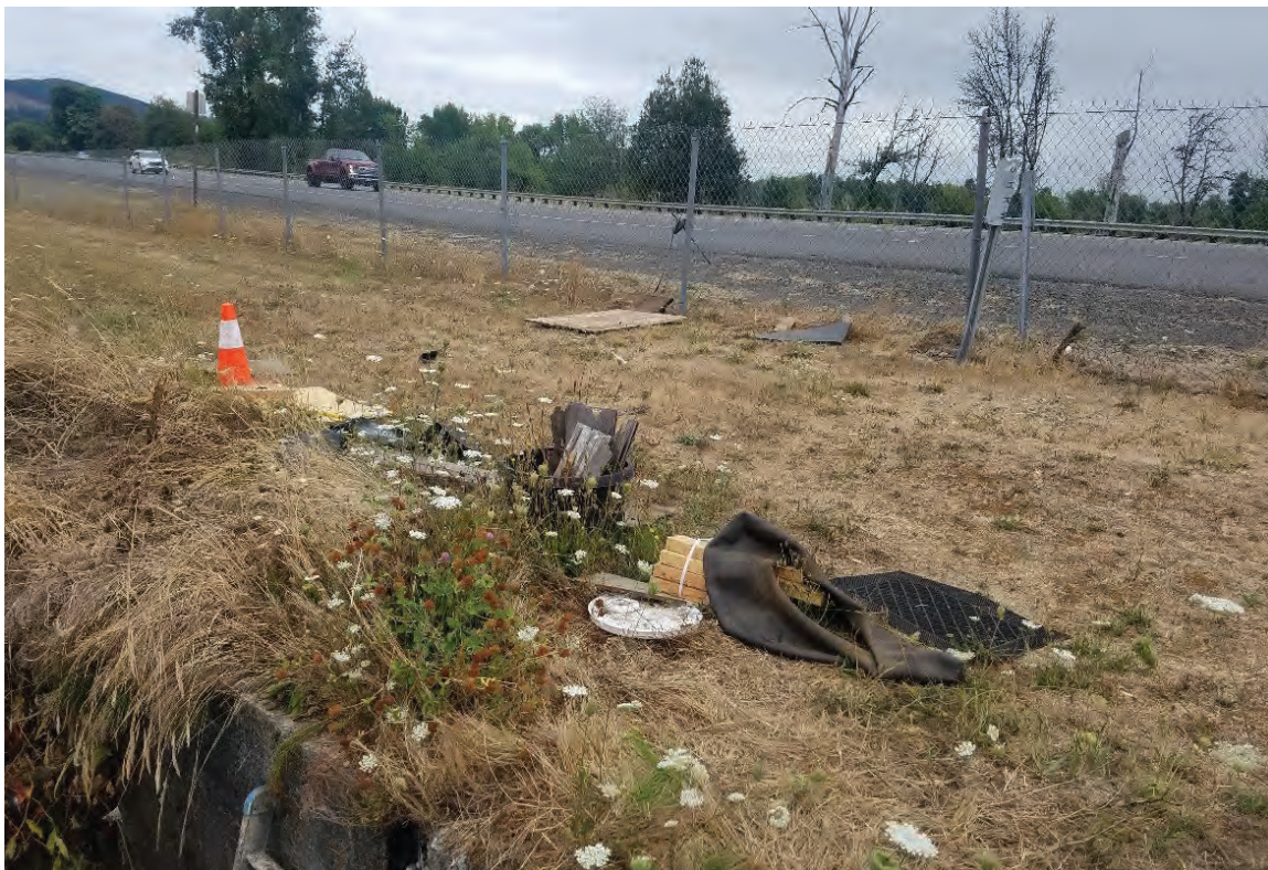
Figure 14: View of the fence and Highway 30. The water control structure is in the bottom left of the photo.
