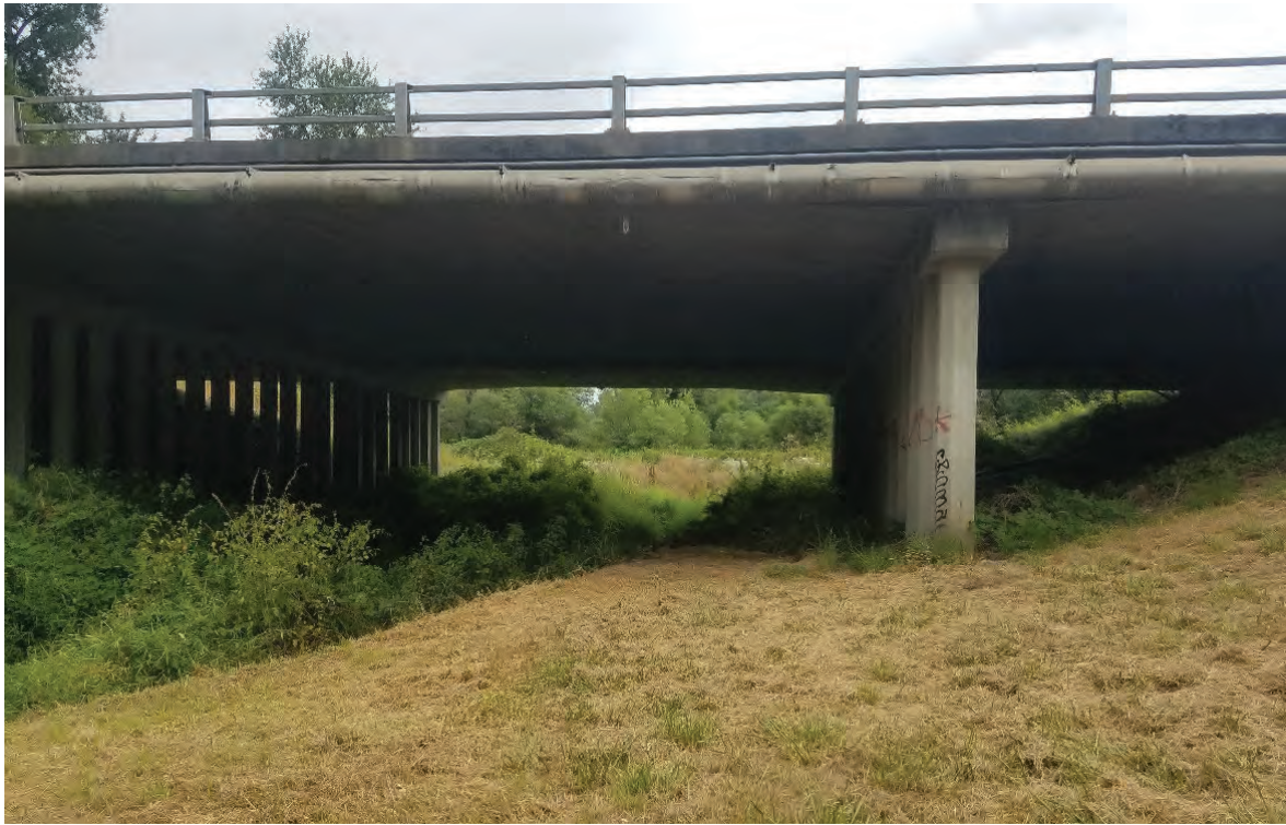
Figure 17: View of the crossing under Highway 30. Wet and dry passage provided here. There are other areas along Highway 30 where a crossing like this one is needed.
