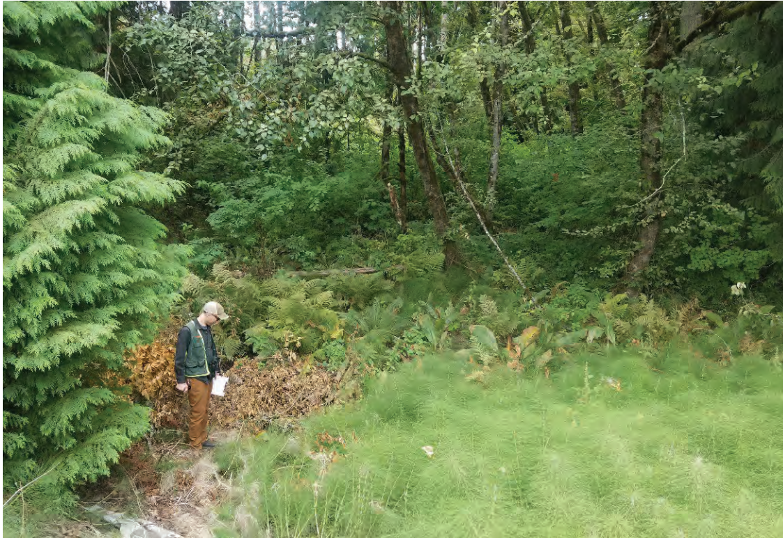
Figure 9: Riparian conditions at a culvert crossing north of the Wildwood Golf Course along Highway 30. Culvert presents a barrier to wildlife crossing.
